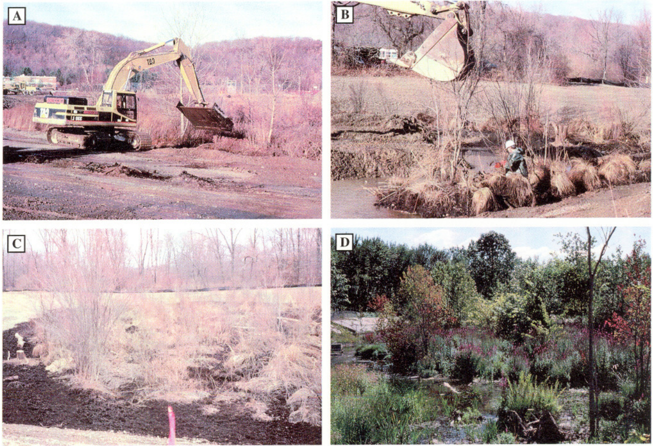
Figure 3. Blanding's turtle habitat restoration, Dutchess County, New York. (A) Sod removal from the donor wetland, December 1996; (B) and (C) Sod placement in constructed wetlands, November and December 1996; (D) Completed constructed wetland, September 1997. (Photos by EK, Hudsonia, Ltd.)
