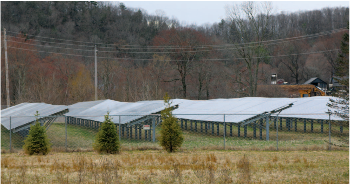
Solar farm in western Massachusetts. Erik Kiviat © 2019
