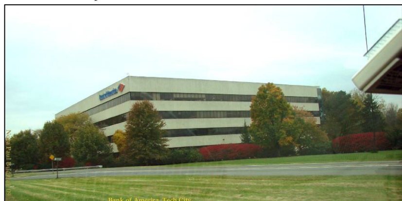
Figure 33: Bank of America in Tech City - Photo by Nora Budziak
